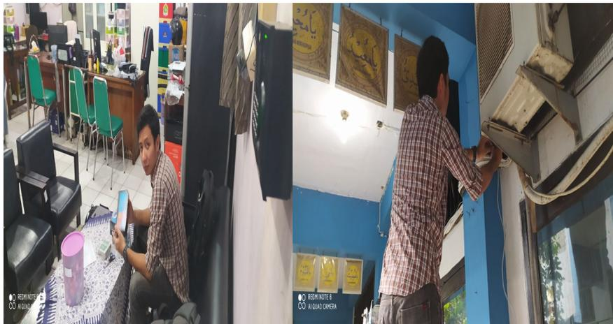
Gambar 7. Instalasi Wireless Distribution Sistem
