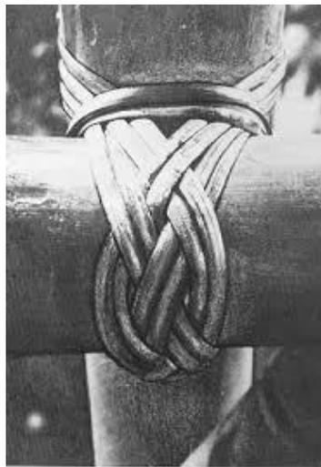
Gambar 1.2. *Friction-tight Rope Connection* [1]
