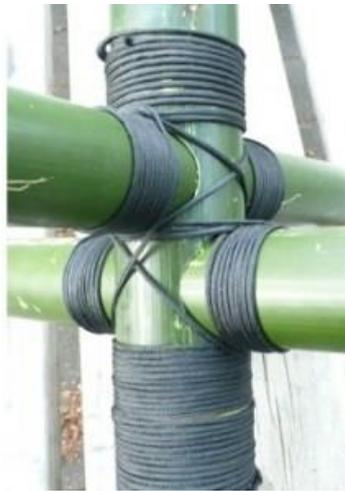
Gambar 1.4. *Interlocking connections* [1]
