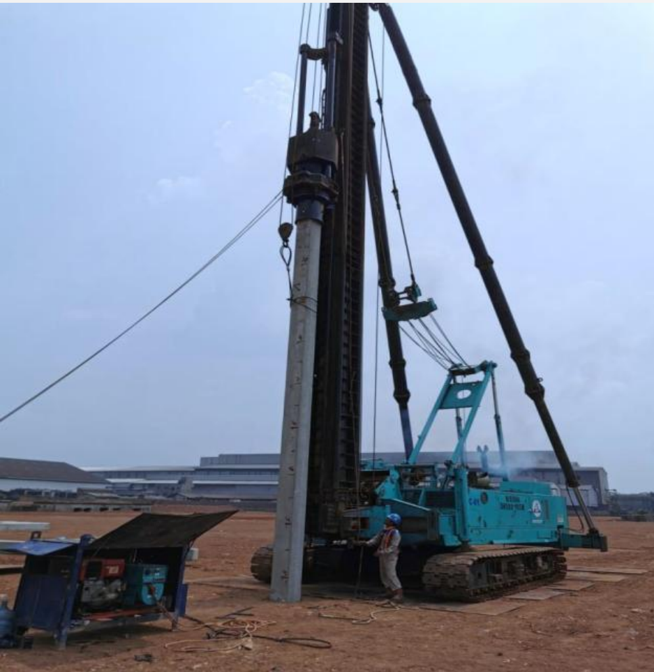
Piling The First Indicator Pile 22 nd Nov 2019
