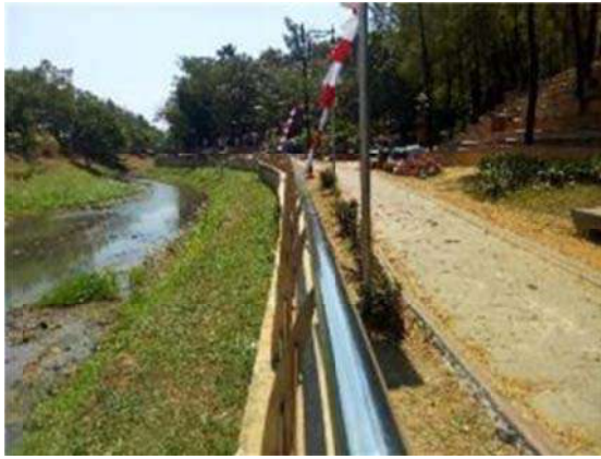
Gambar 1.8 Jalur Jogging Track di Jaletreng River Park, Tangerang Selatan (Sumber: Aprillia dkk, 2020: 239).
