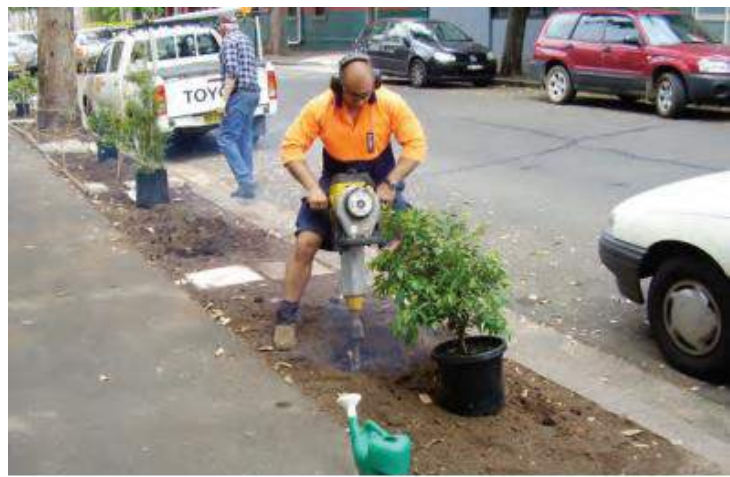
Council worker using jack hammer to excavate dead soil, toughened by years of no water, no nutrients, nothing except people walking over it.
