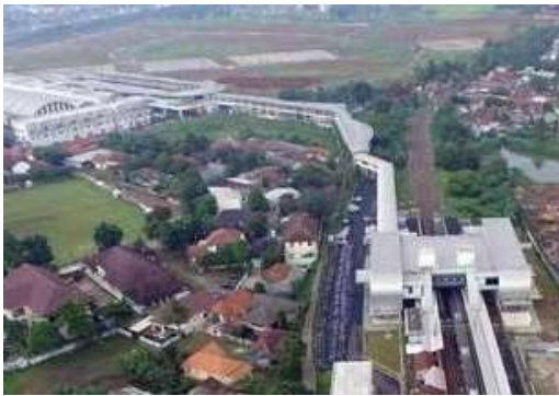
Figure 8 Skybridge. Source: StasiunCisaukjadipeluangemaspengembang, Dwytia Putra, 2019
