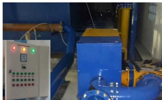
Figure 4. Micro-hydro installed in water treatment plants
