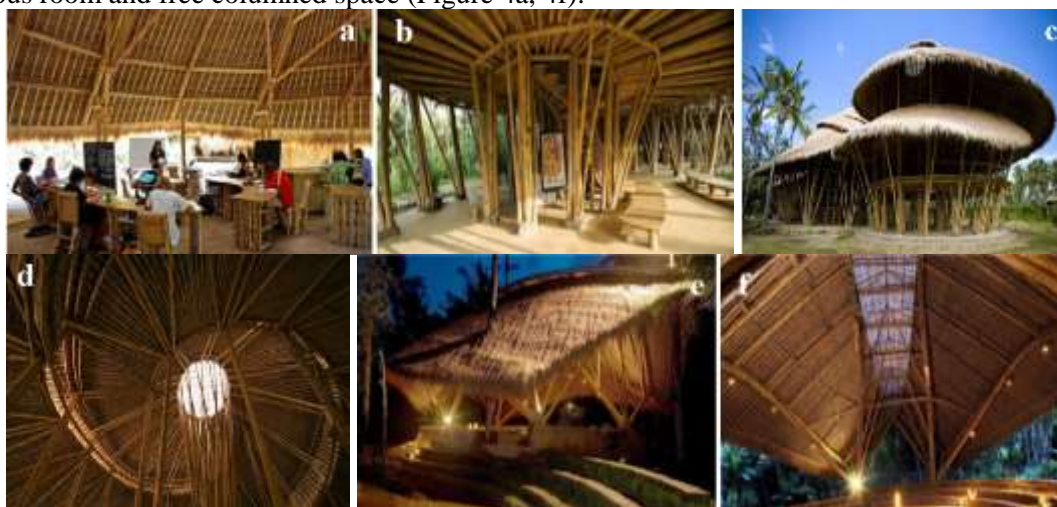
Figure 4. Green School Used Bamboo Material for Construction and Finishing
