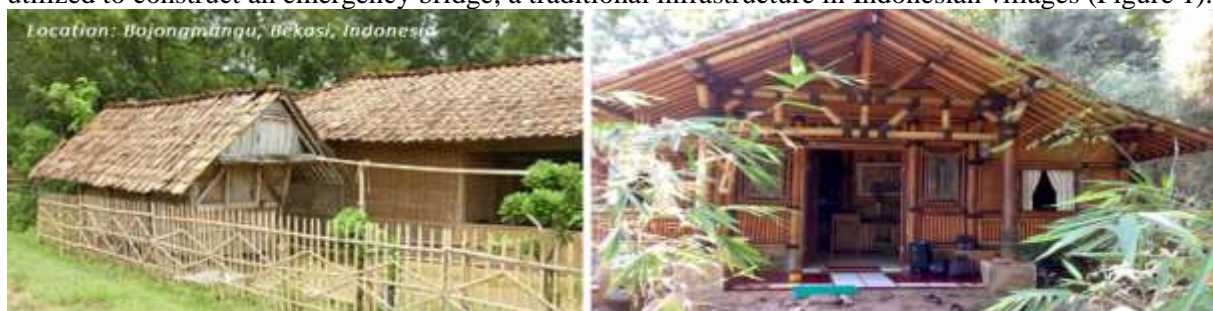
Figure 1. Construction of Bamboo Fences, Walls, Column and Roof Truss.
