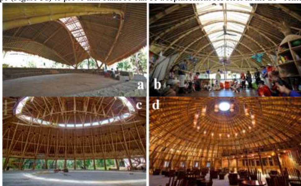
Figure 5. Bamboo Material for Wide Span Building Construction
