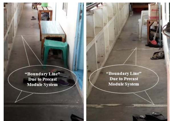
Fig. 1. Precast module system on corridor. Surveyed on August 16, 2016.
