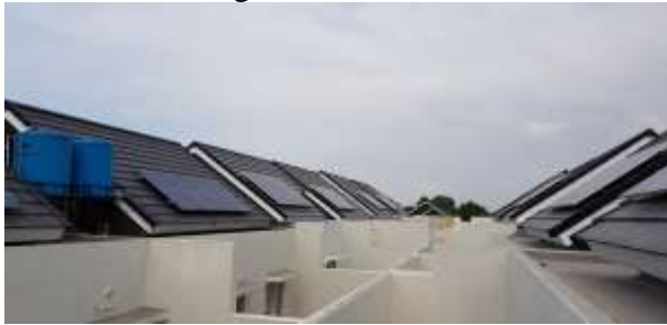
Figure 10: Solar Panel installation Source: Private documentation, 2019
