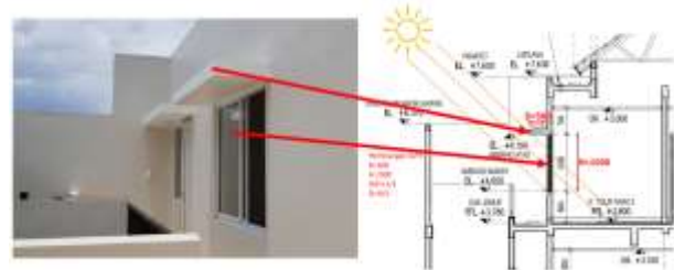
Figure 8: Shading devices that is not efficient Source: Private documentation, 2019
