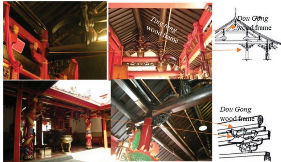
Figure 8. The wooden roof frame structure of the Dou Gong and Ting Tang on “Kelenteng Hok Tek Bio”.
