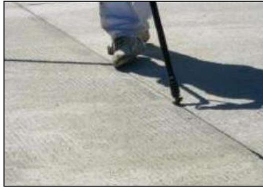
Gambar 2.35. *Joint and crack sealings*
