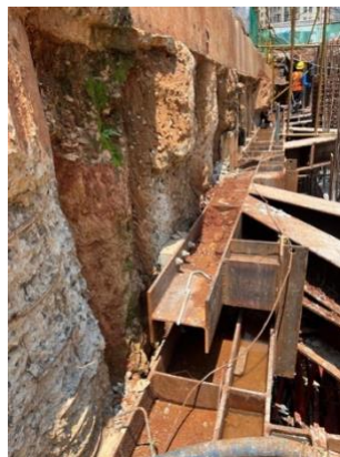
Gambar 1. Waler Beam dan strutting
