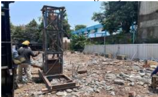
Gambar 7 Pelaksanaan Pile Driving Analyzer Test
