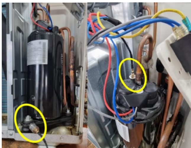
Fig. 6. Vibration sensor location
